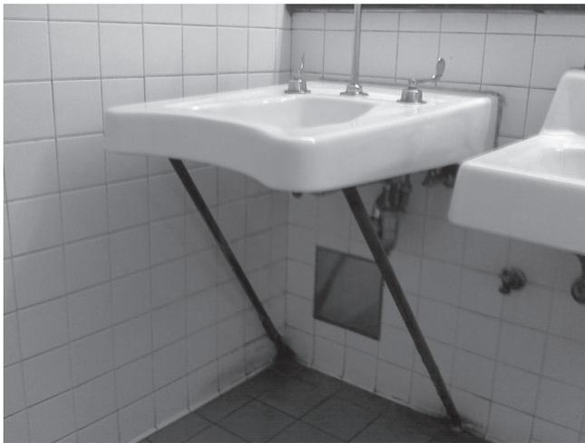
It appears the wall hung lavatory became loose from years of public use. Instead of fixing or replacing the concealed arm carrier in the wall, the solution was simple. Someone cut two wooden poles to length and wedged one end in the arm carrier holes on the underside of the lav. The other end fit snugly in the corner where the floor and wall meet. Problem solved.
